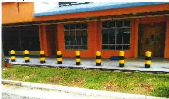
Safety bollards installed in front of a childcare centre.
