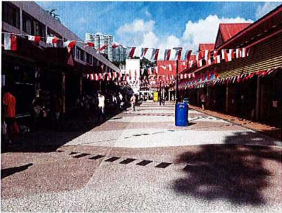
Granolithic flooring coated on Blk 338 Ang Mo Kio Ave 1 open space
